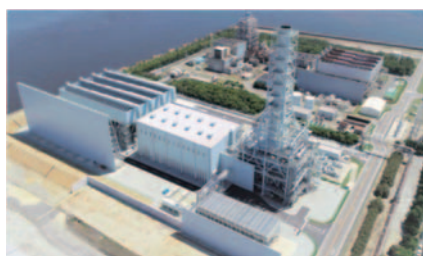
Fig. 24 The new pilot plant (T-point 2) of M501JAC gas turbine (7)
