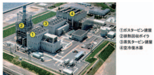
Fig. 20 Gas turbine combined cycle power generation plant demonstrator (T-Point) (5)
