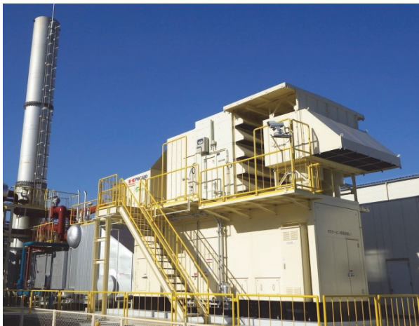
Fig. 21 Gas turbine generator set on assembling
