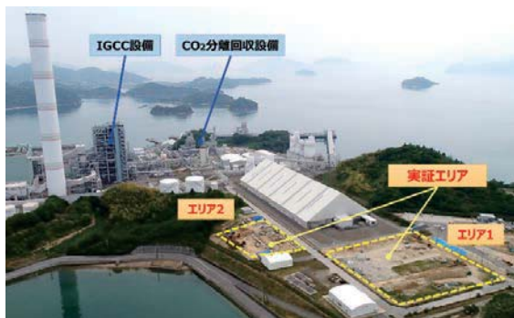
Fig. 17 Demonstration area for effective use of CO 2
