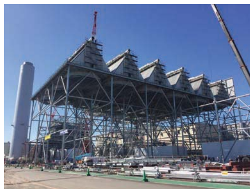
Fig. 8 No.1 ACC under construction
