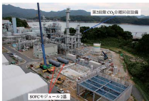
Fig. 16 Third step construction status (August, 2021)
