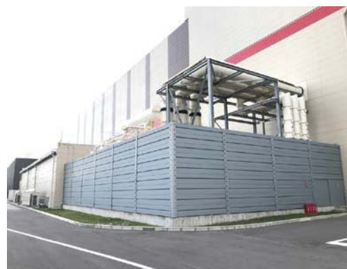
Fig. 10 Gas turbine transformer
