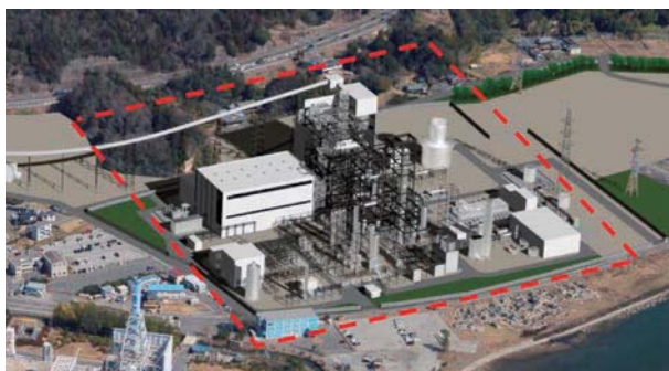
Fig. 8 Bird's-eye view of Nakoso site
