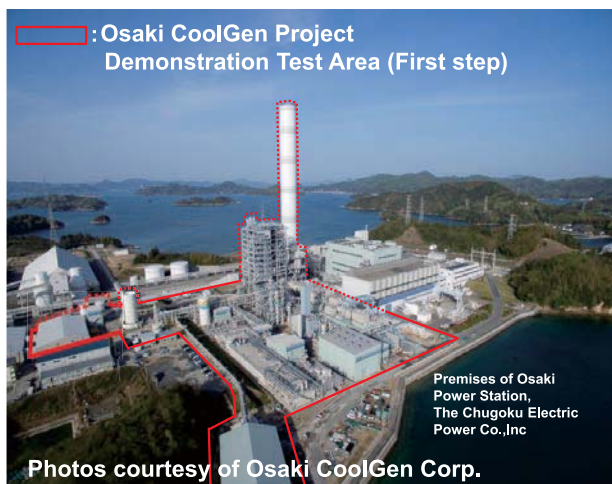
Fig. 11 Bird's-eye view of Osaki CoolGen project
