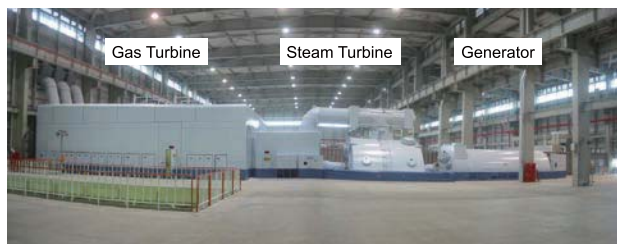
Fig. 2 Example of gas turbine combined cycle
