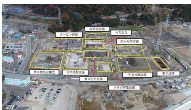
Fig. 10 Construction status of Nakoso site (6)
