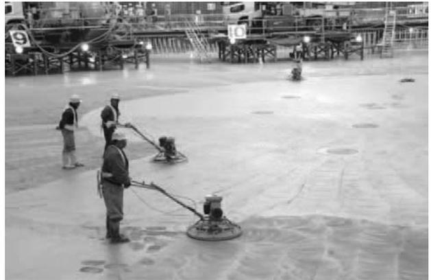
Fig. 5 Surface leveling of placed concrete
