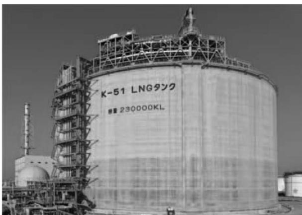
Fig. 15 Overview of 230,000m<sup>3</sup> PC LNG tank in Senboku LNG Terminal 1, Osaka Gas
