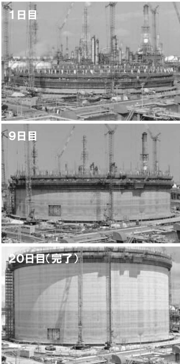
Fig. 14 Result of slipforming construction
