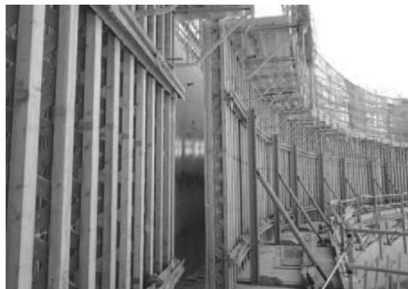
Fig. 4 Formwork and scaffolding system
