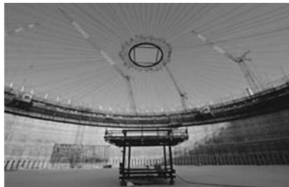
Fig. 12 Spoke wires (the adjustment mechanism)
