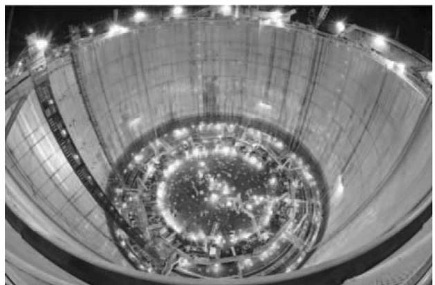
Fig. 7 Cylindrical slurry wall
