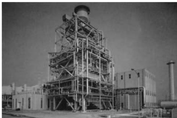
Fig. 7 Heat recovery steam generator
