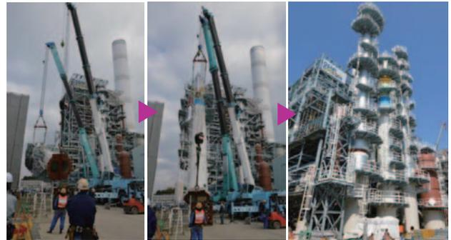
Fig.12 Transportation of Gas cleanup unit
