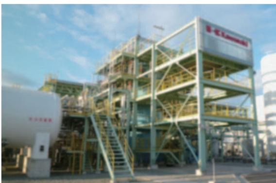
Fig. 3 Hydrogen liquefaction system
