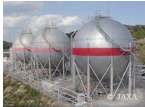
Fig. 4 Liquefied hydrogen storage tank
