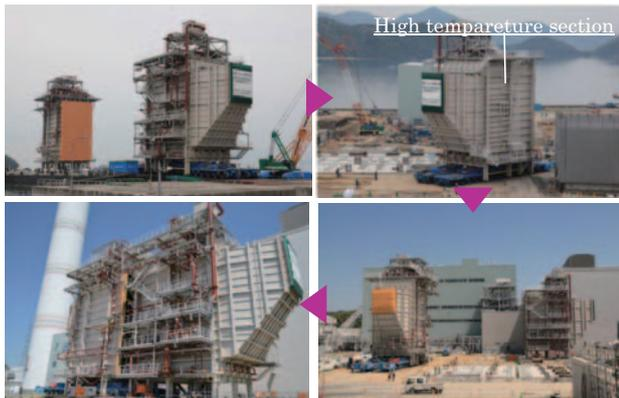
Fig.15 Transportation of HRSG
