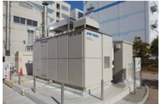
Fig. 3 The appearance of 100kW PAFC (FP-100i)
