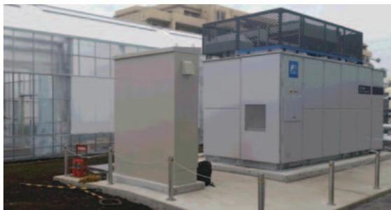
Fig.12 100kW PAFC for emergency use and vegetable plant
