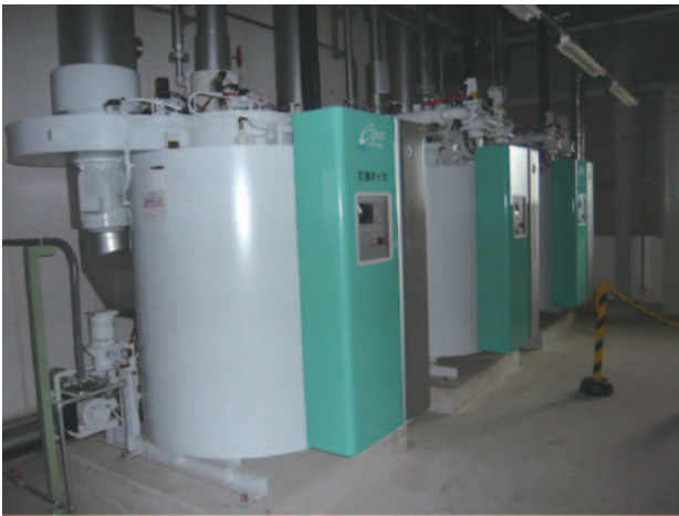
Fig.12 Biomass boiler
