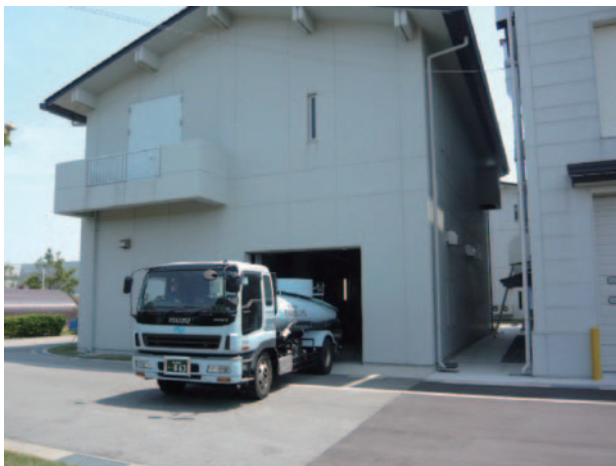
Fig. 6 Delivery entrance of digested sludge
