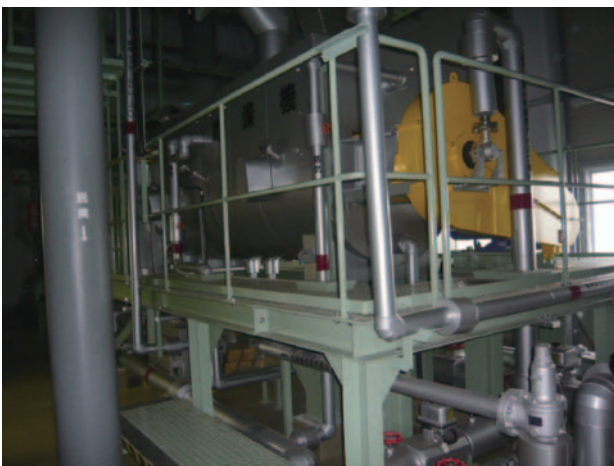
Fig.13 Sludge dehydrator
