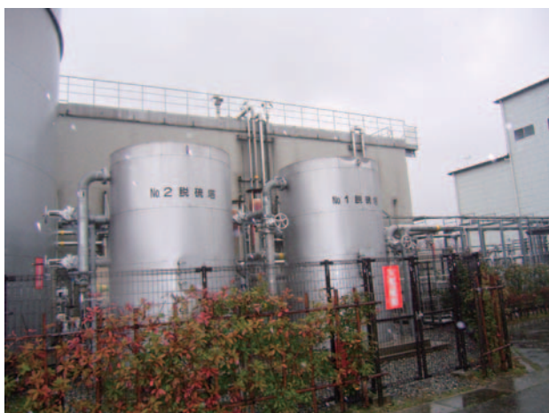
Fig.10 Desulfurization equipment
