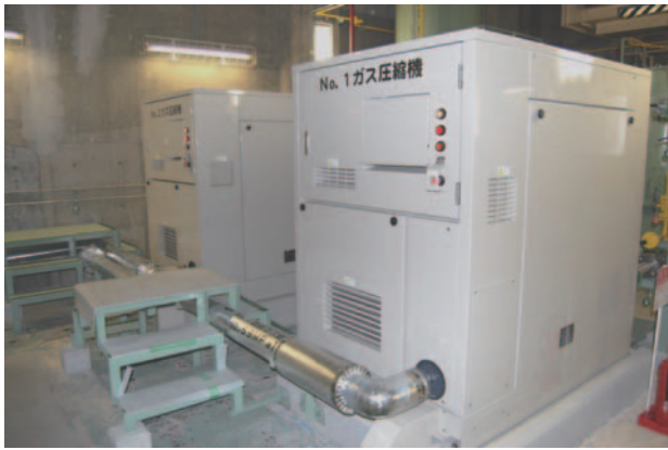
Fig. 4 Gas Compressor
