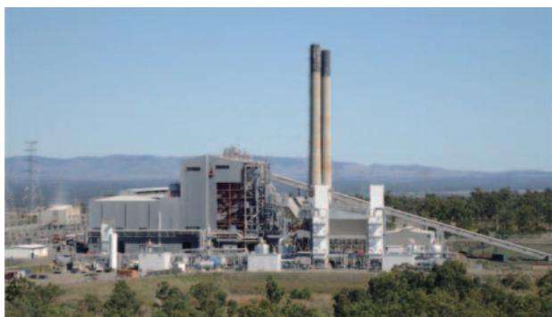
Fig. 8 General view after modification
