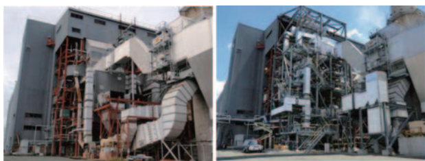
Fig. 6 Before (left) and after (right) the modification
