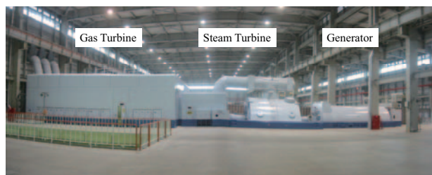
Fig. 5 Example of gas turbine combined cycle
