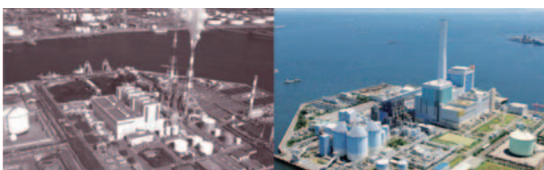
Fig. 4 Old and New Isogo Coal-fired Thermal Power Station
