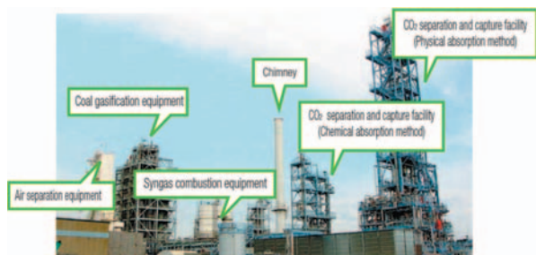
Fig.11 External View of EAGLE Pilot Plant test facility
